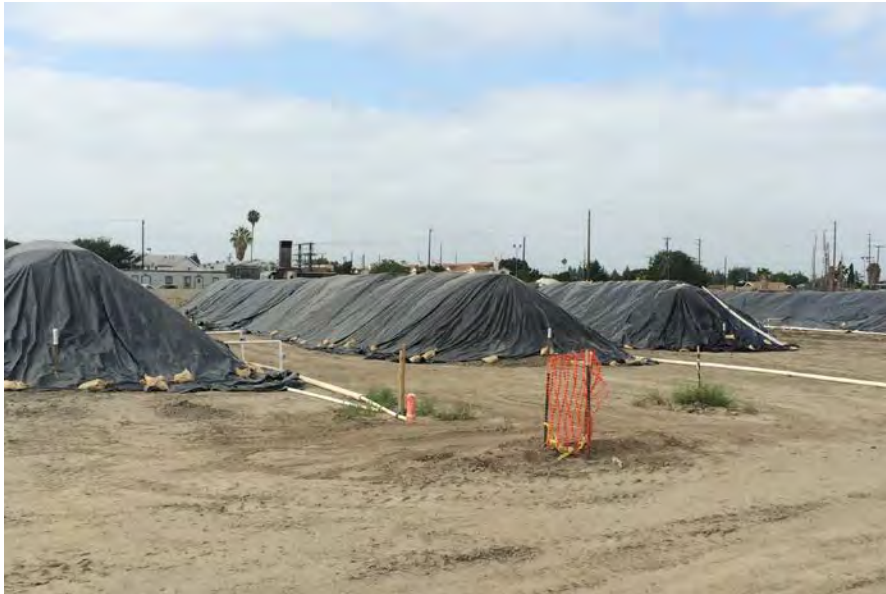
Photo 5: Treatment soil piles.
