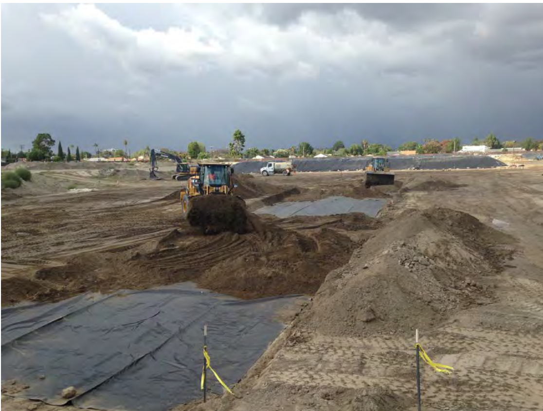
Photo 4: Treatment soil pile construction in former Basin 80013.
