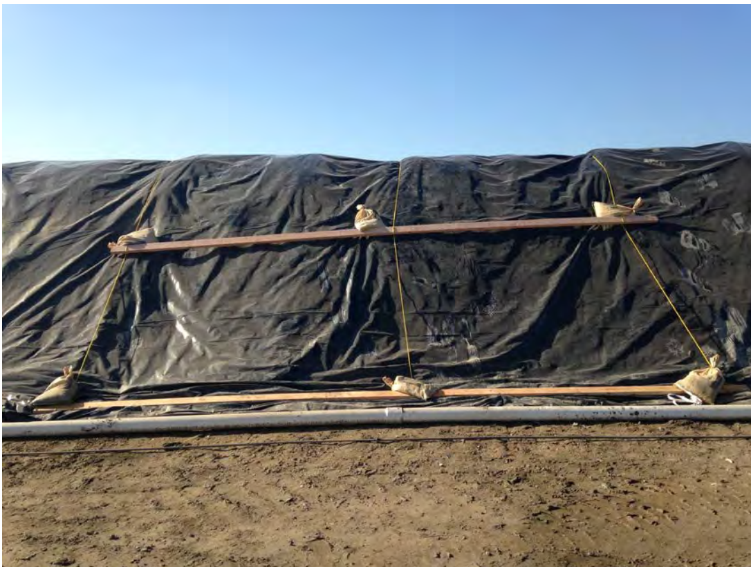
Photo 2: Soil treatment pile cover management.
