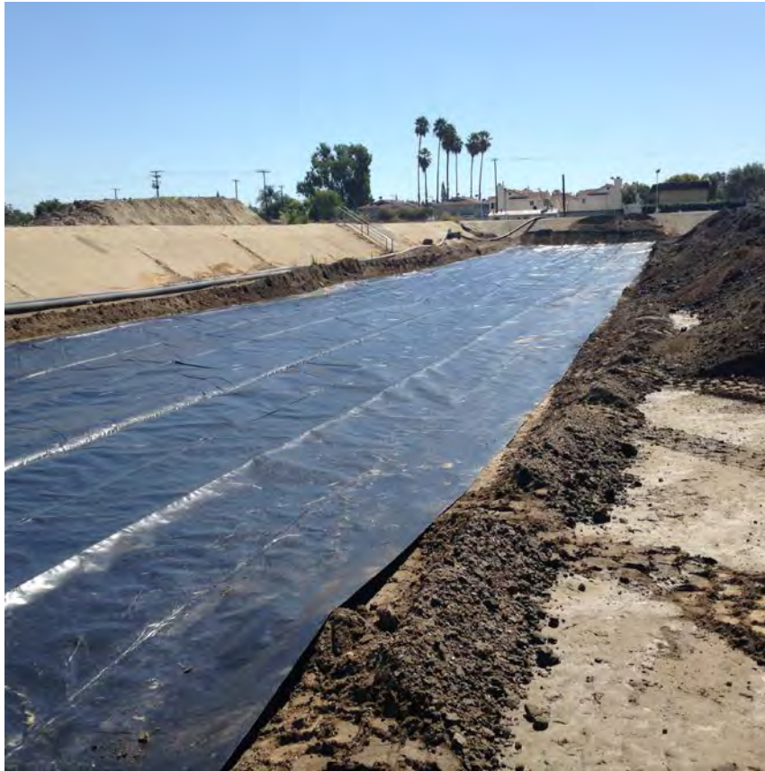
Photo 3: Treatment Soil Pile construction in former Basin 80013.
