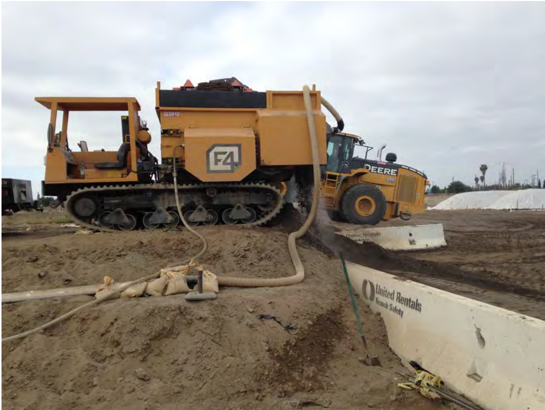
Photo 1: Bulldog Green Remediation, Inc. equipment.
