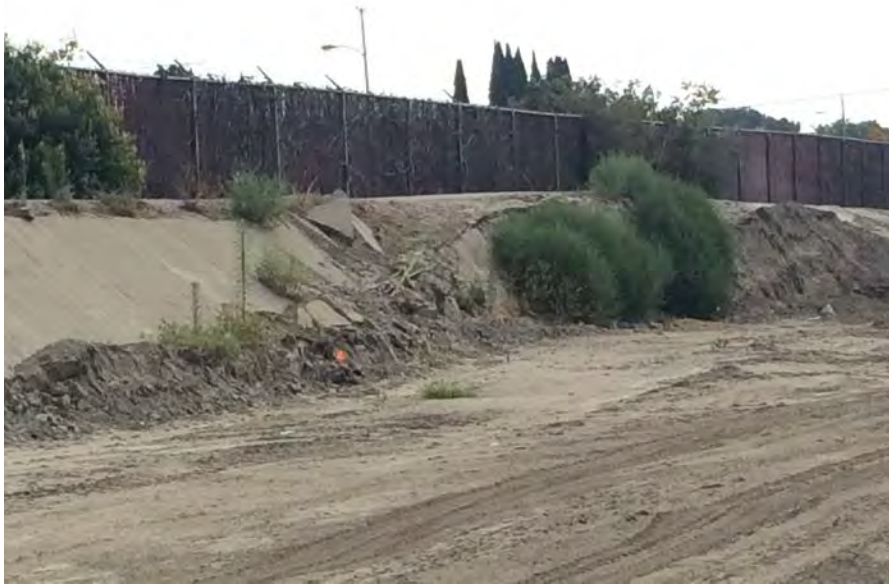
Photo 9: Berm along northern edge of site that prevents runoff.
