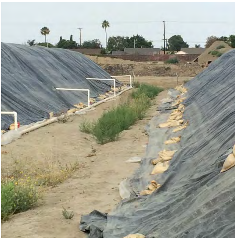
Photo 8: Drainage feature between soil treatment rows for runoff control.
