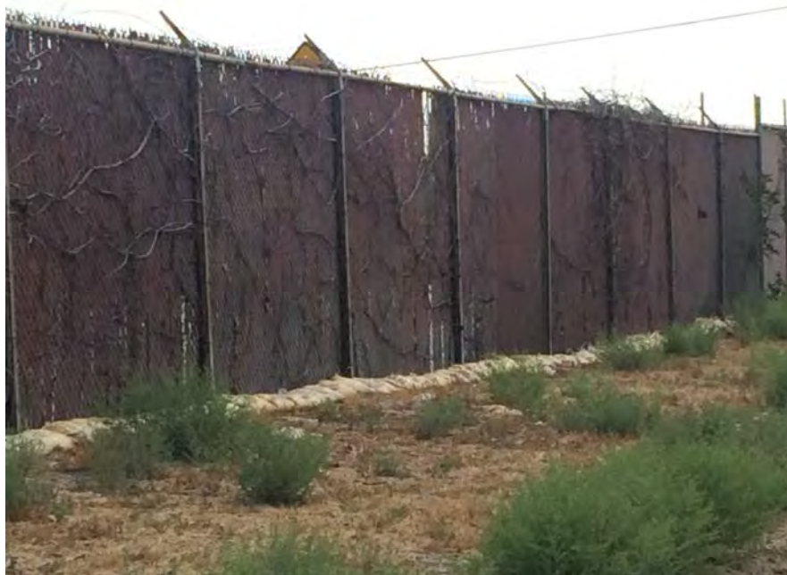
Photo 10: Perimeter sandbags to prevent runoff.
